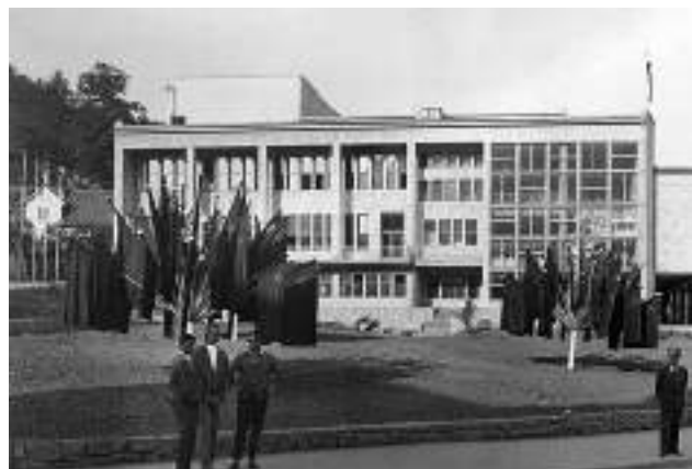
Cultural center Delavski dom Zagorje (Source: KCDDZ)
